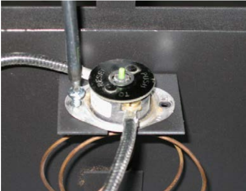
Unscrew Hi-Limit from frame
