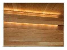
Fabricated using two pieces of 1x4 t & g. Rip tongue off one piece and the groove off the other. Glue the two boards together.
