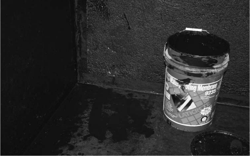
Waterproofing treatment of corner and floor with LATICRETE® 9235 Waterproofing Membrane.
