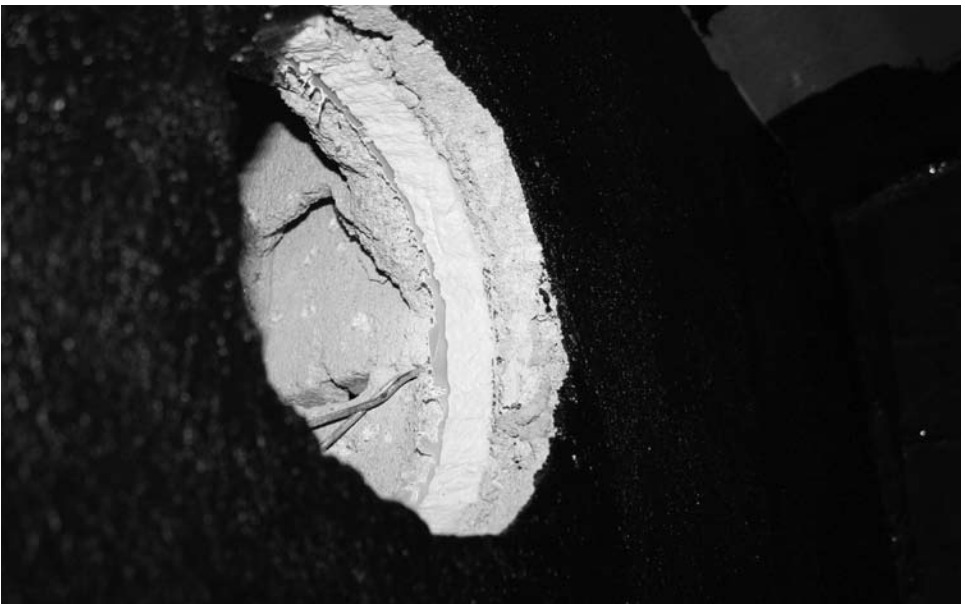
Lighting fixture waterproofing membrane pre-treatment. The vapor retarder, insulation board, mud bed, and LATICRETE 9235 Waterproofing Membrane are all clearly visible.
