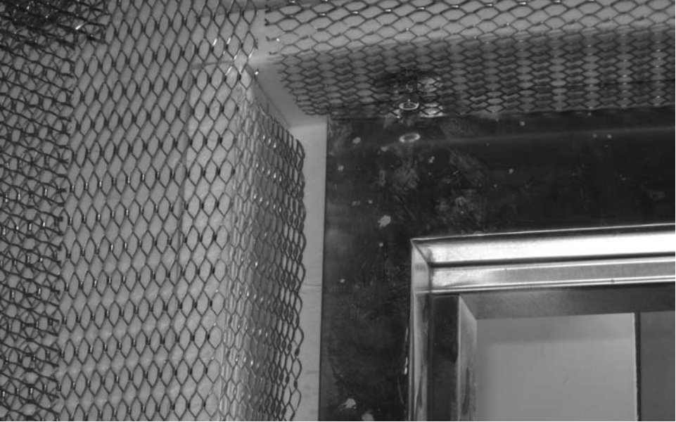
Installation of 3.2# expandable diamond metal lath to stainless steel door frame and flashing.
