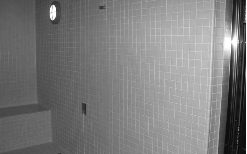
Finished wall showing door, light and emergency call switch installations.
