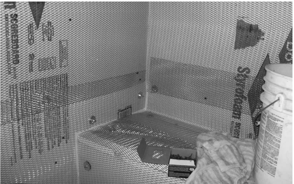
Bench/wall transition and proper placement of 3.2# expandable diamond metal lath.
