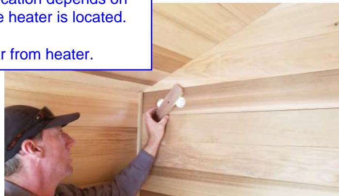
Install the cedar vent cover over the outlet holes on the inside of the sauna with a 1 1/2" screw.
