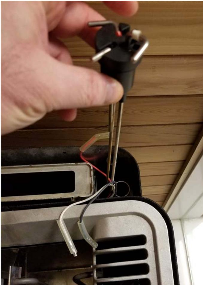
**Carefully slide wire connectors off electrodes
