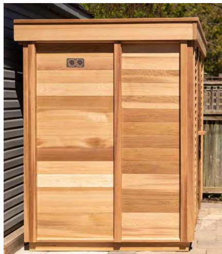
Outlet vent high on opposite wall of heater.
