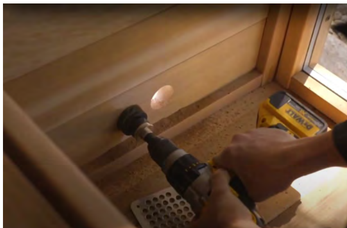
Inlet holes drilled under electric heater on side wall
