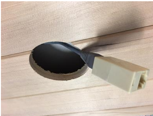
CAT-5 with in-line coupler attached
