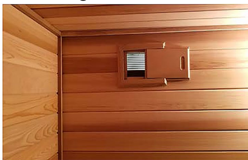
High on the wall
