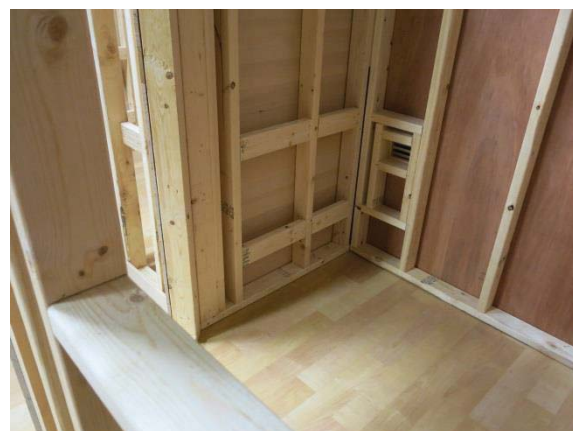
Photo 02. Notice bench support blocking and location of upper vent.
