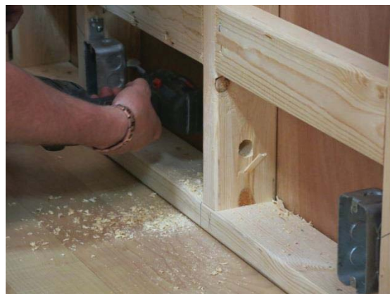
Photo 05. Drill 7/8" diameter holes for your MC/BX cable.
