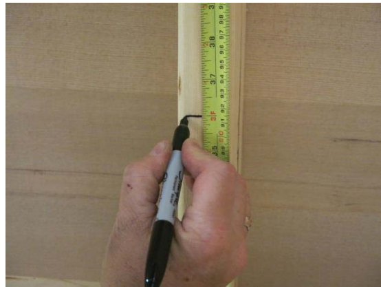
Photo 03. Marking the height of the IS panels.
