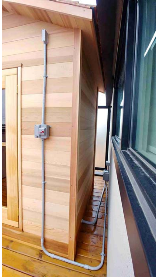
Weather proof conduit & light switch i.e. solid log Cabin or Barrel sauna
