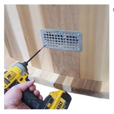
Install 1 of the stainless steel vent grills on the outside of the sauna centered over the holes using 1 ½" screws. (6pcs)
