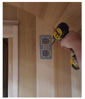
Install Stainless Vent cover on the outside using 1-1/2" stainless steel screws. (6pcs)
