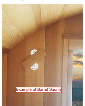
Install the cedar vent cover on the inside of the sauna with a  $1 \frac{1}{2}$ " screw.
