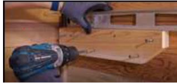
Cedar cleat (with kit) mounts through cedar lining into blocking.
