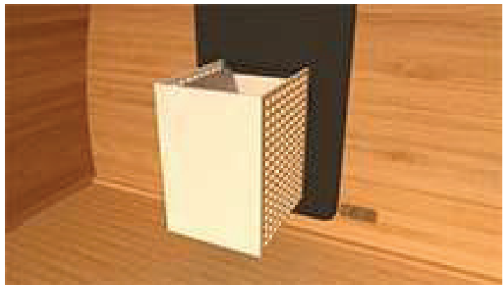
Inlet beside wood heater on Back wall
