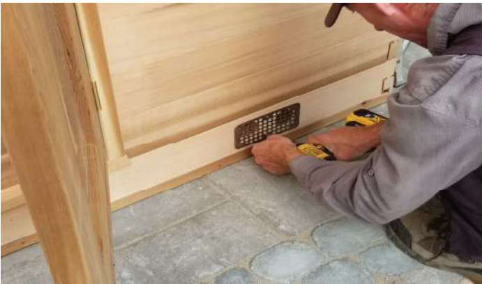
Install 1 of the stainless steel vent grills over the inlet holes on the outside of the sauna centered over the holes using 1 1/2" screws. (6pcs)
